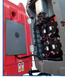
Compartment des batteries
